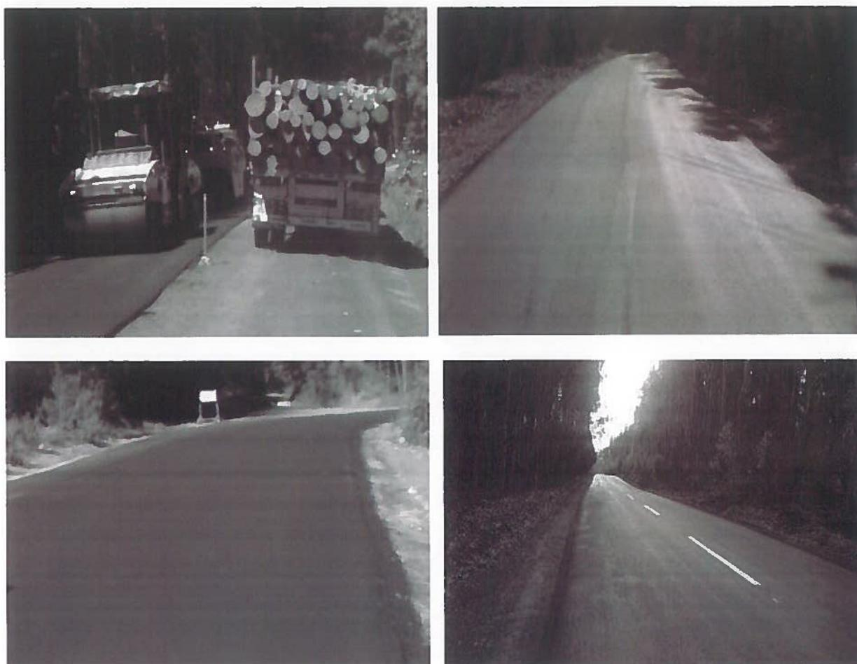
**FOTOS 13: BASE PROES CON MEZCLA ASFALTO EN CALIENTE, ESPESOR 4,0 cm**
