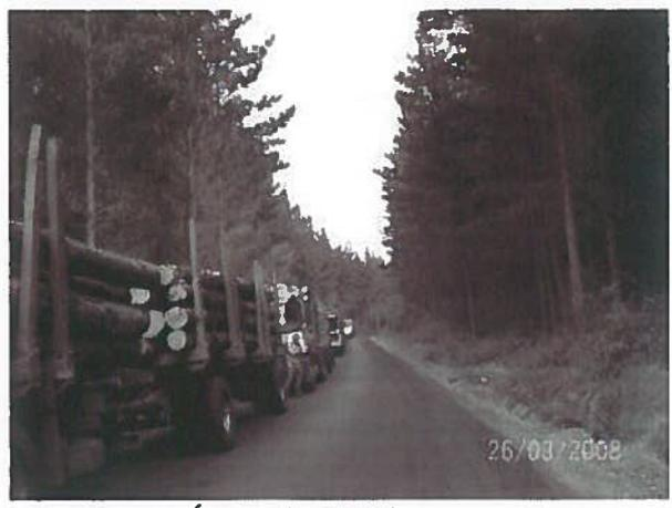
FOTOS 11: BASE PROES CON TRATAMIENTO ASFÁLTICO (SLURRY)
