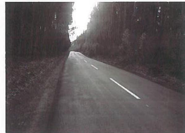
**FOTOS 13: BASE PROES CON MEZCLA ASFALTO EN CALIENTE, ESPESOR 4,0 cm**
